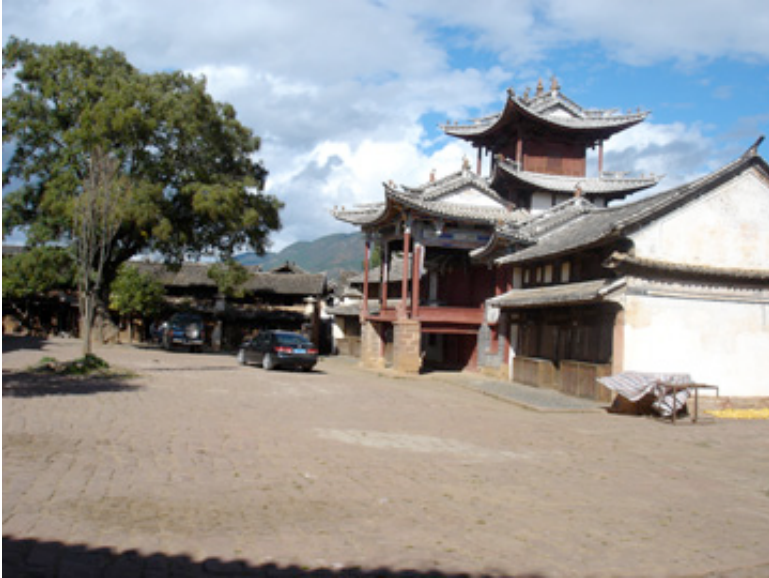
Shaxi Rehabilitation Project
